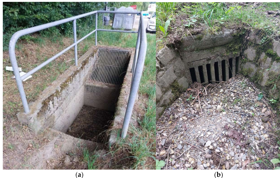
Figure 2. Examples of (a) a two-dimensional screen (screen number 17) with a silt trap; and (b) a one-dimensional screen (screen number 21) without silt trap after heavy rain (May 2024) in Oberstedten, Oberursel (Taunus).
