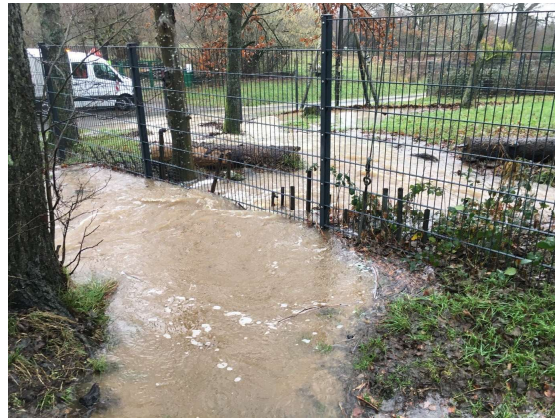
Figure 1. Example of flooding of a street, path, and private property due to blockage of a screen (screen number 4) and a pipe during heavy rain (January 2023) in Oberstedten, Oberursel (Taunus).
