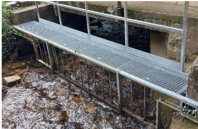
Figure 6. Example of a pre-screen (screen number 26) protecting a main screen (screen number 25) further downstream.
